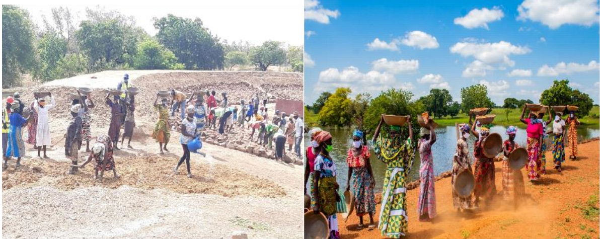
Formation of Embankment of Small Earth Dams by Beneficiaries
